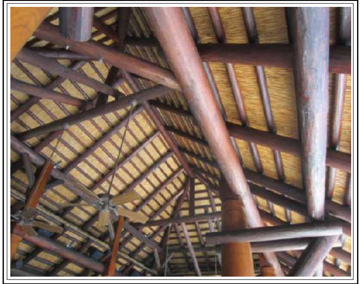
Natural roofs on exterior buildings
