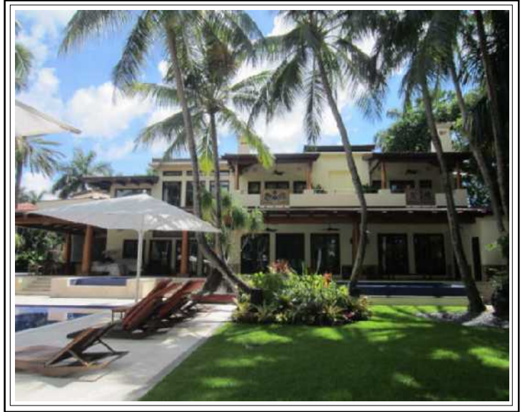
Main residence rear view
