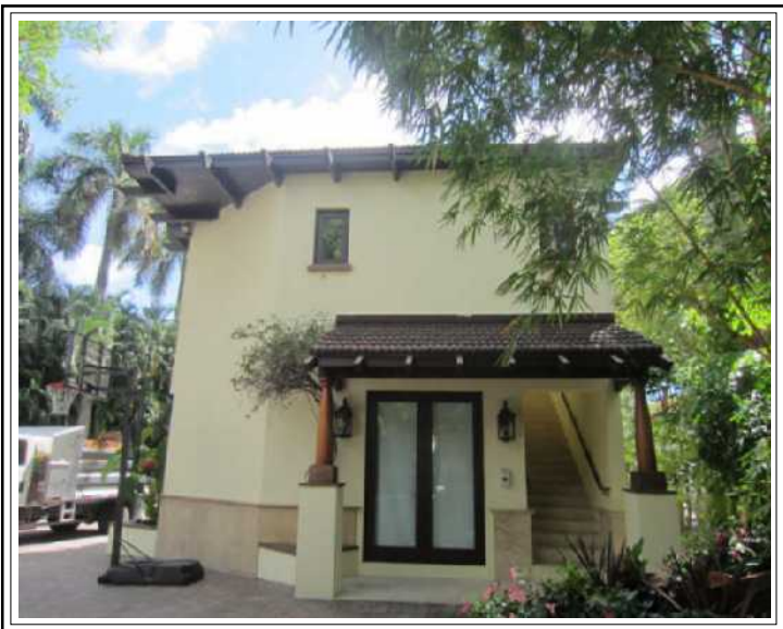
Front guest house side view with stairs
