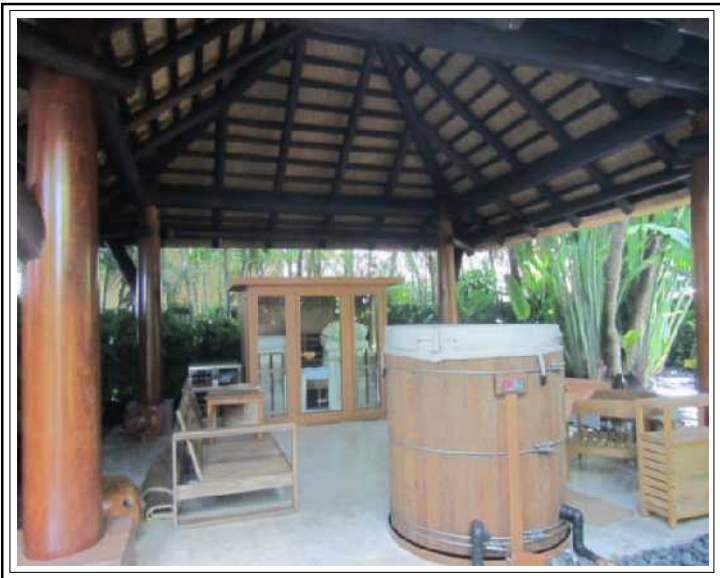
Natural roofs on exterior buildings
