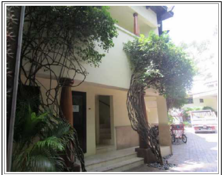
Front guest house first floor entry
