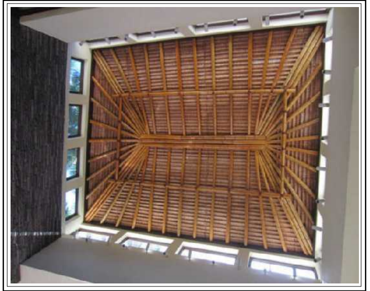
Natural roofs on exterior buildings
